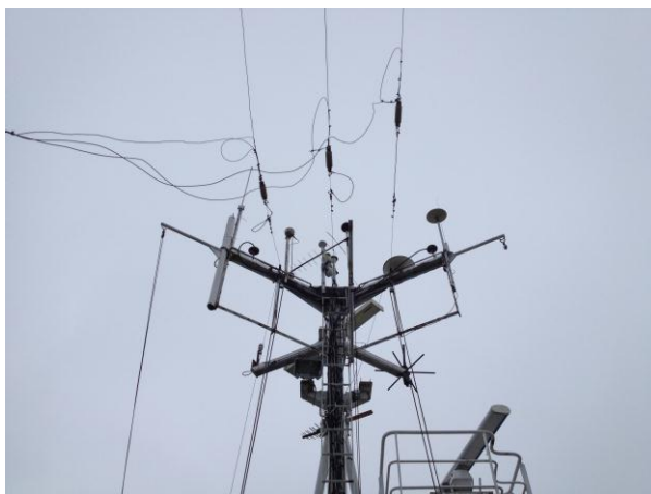
Figure 4: GNSS Antenna Mounting Arrangement
