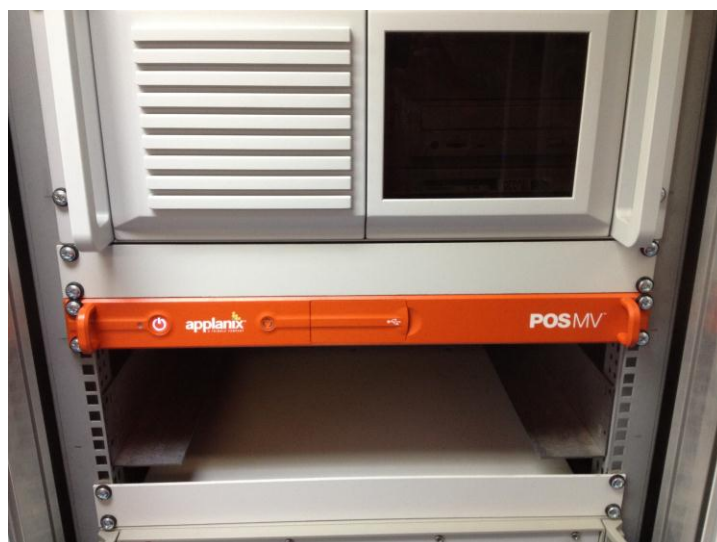
Figure 2: POS MV PCS Installation Location
